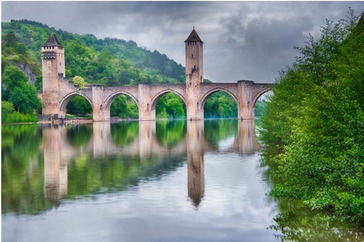
The ancient fortified Pont Valentre in Cahours.
